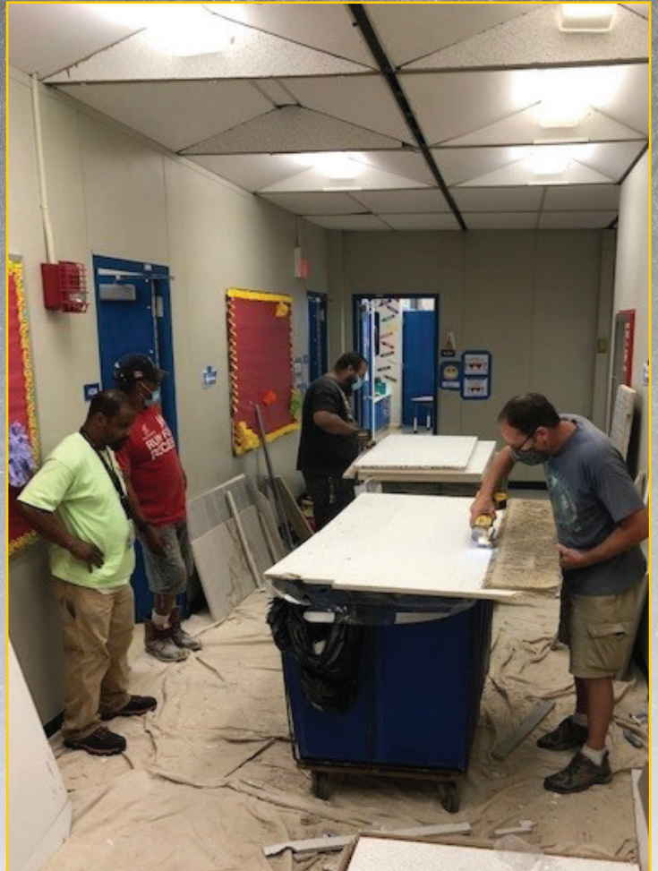
Members repair ceiling tiles.
