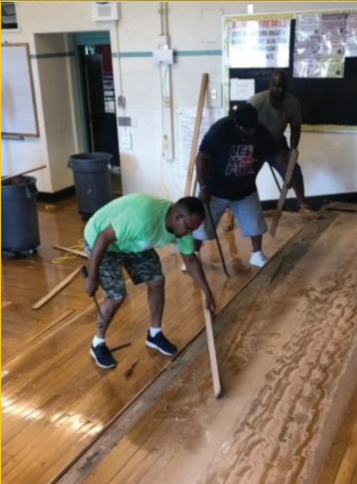
Floor work at BLA.
