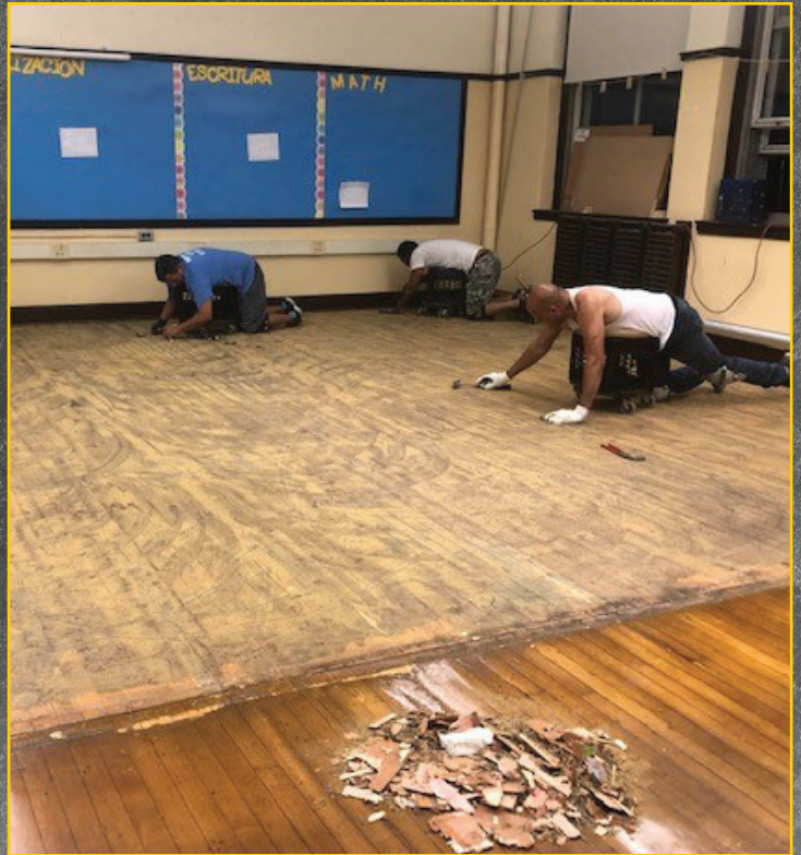
Members repair the floor at Boston Latin Academy.
