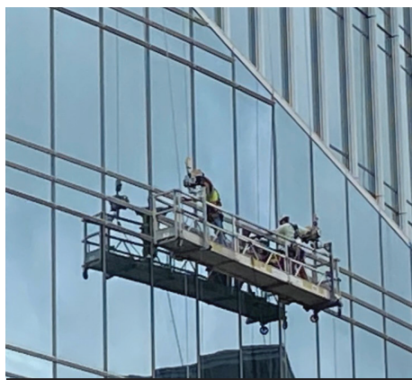
Local 1044 Glaziers Greg Leonard and Mike Pickup Sr. swing the unitized curtain wall at 1 Congress Street. Sometimes the $1.00 an hour premium just doesn't seem like enough.
