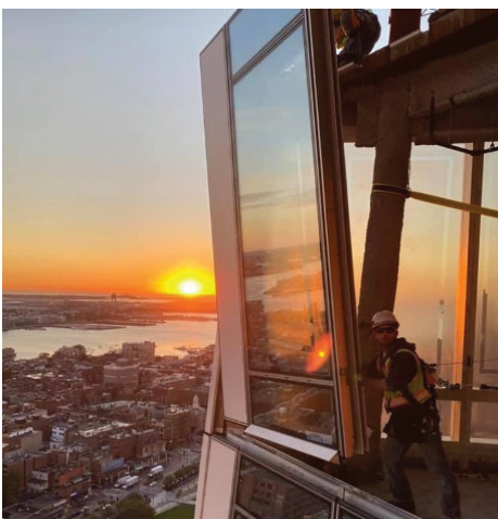
Local 1044 Glazier Peter Drohan guides in a glass panel at 1 Congress Street in Boston for Benson Industries.
