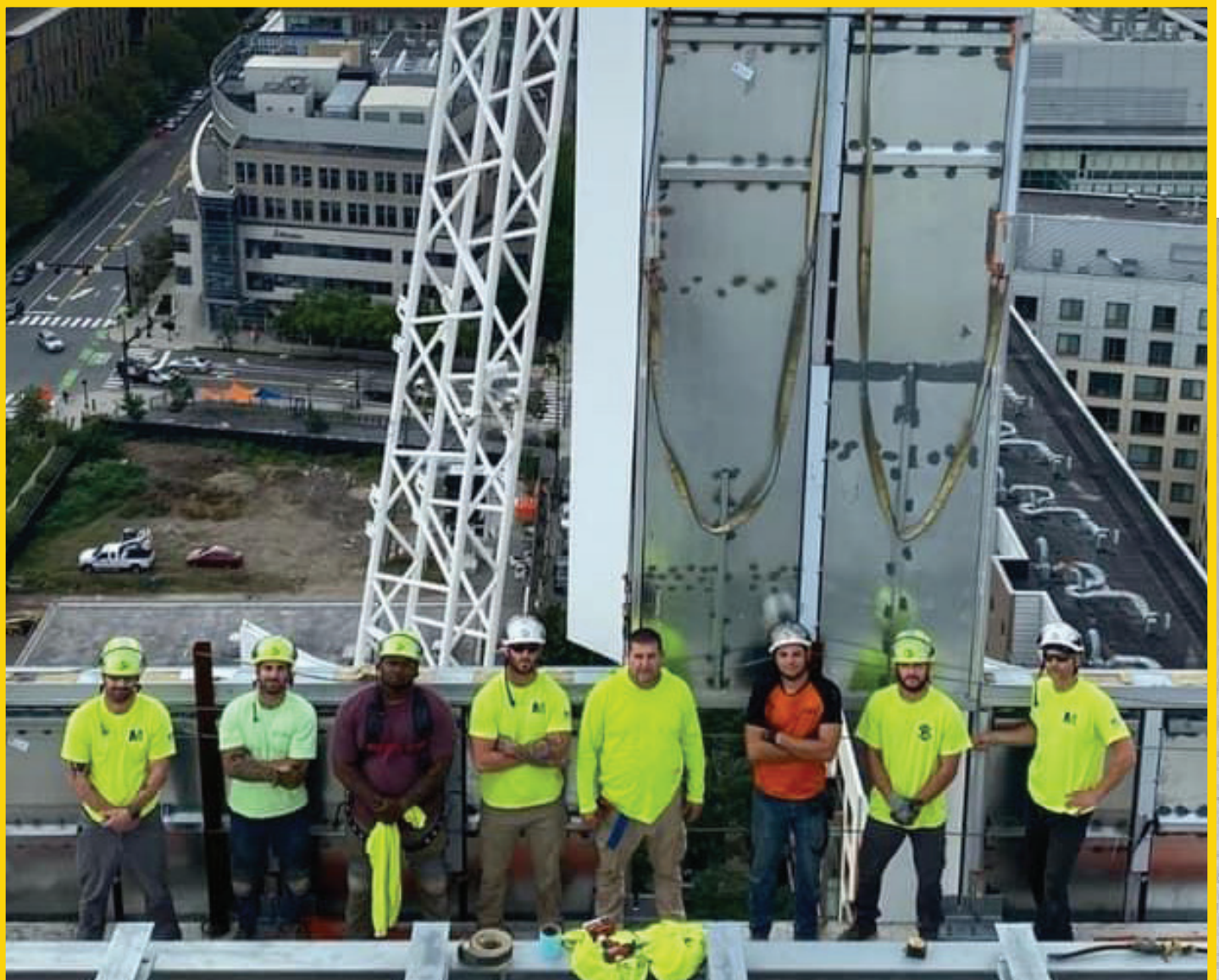
DC 35 members hard at work at high-rise job site.
